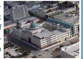
Aerial view of City Hall
