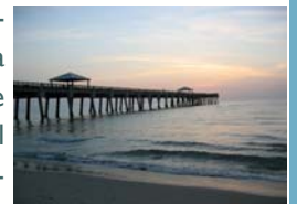
Production Photo of the Juno Beach Park & Pier
